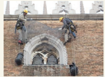
Detail of the precautionary operations on the large windows, carried out with qualified restorers at work in rope
