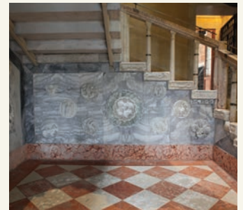
Overall view of the main staircase
