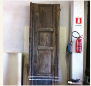
Front view of a door with an indication of the cut to be made for rehabilitation
