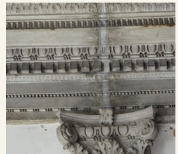
Detail of the morphological degeneration of the stone surfaces
