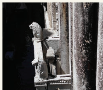
Detail of one of the balconies made of Istrian stone
