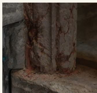
Detail of a degraded limestone "rosso Verona"
