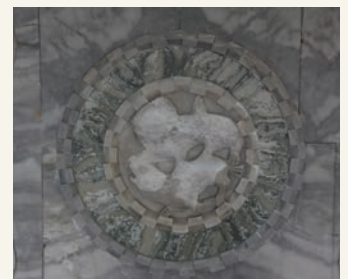
Detail of an ancient crystal marble patera with advanced degradation
