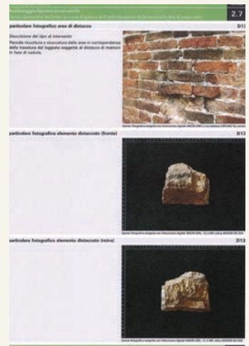
Detailed study of conservative critical issues on the façade
