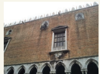
View of the façade during the inspection and safety measures carried out with qualified restorers at work in rope
