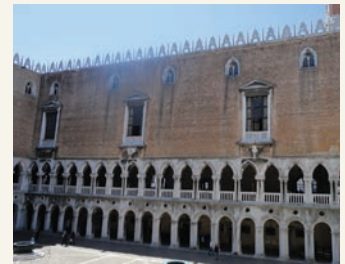
View of the west façade overlooking the internal court
