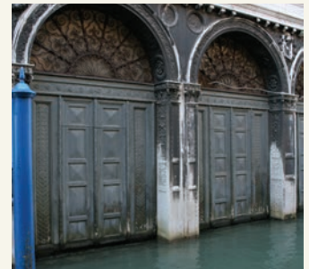
Wooden nineteenth century doors before the dismantle for the restoration in 2007
