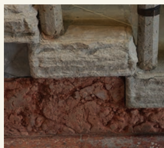
Detail of a degraded limestone "rosso Verona"
