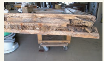
Bottom View of the doors, the degradation of the wood is visible due to the attack of micro - marine organisms
