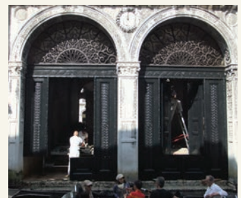
View of the twin gates already restored during their reassemble in place. The new selective opening mechanism of the various parts, resulting from the cut of the lower portions and the insertion of new independent portions, is visible
