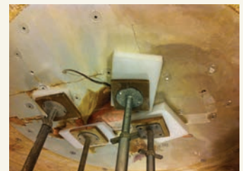
Detail of the central area during the functional supervision of operations to ensure the temporary suspension of the ceiling, which presented subsidence phenomena
